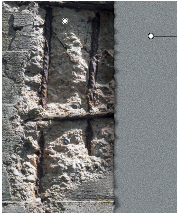
Concrete repairing area
